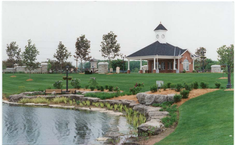
Figure 5.2 - Man-made retention pond landscaped to restore the area in an environmentally sensitive manner and improve water quality through the planting of indigenous plants.
